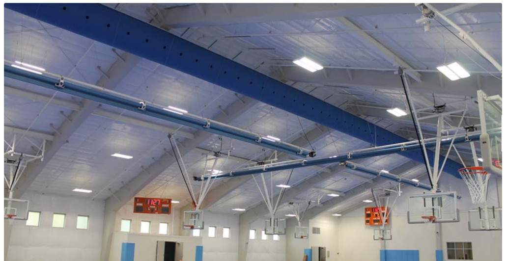
Example of Fabric Duct HVAC System
