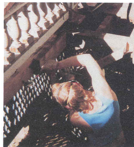
Above: Close ground and poor ventilation kills floor framing first. Pressure-treated lumber (which can hide behind a skirt board) holds up under high moisture. Below: Lifting sections of porch floor gives access for structural repairs. Bottom: A porch is only as level as its piers. Rebuild crumbling footings while the framing rests on cribbing.
