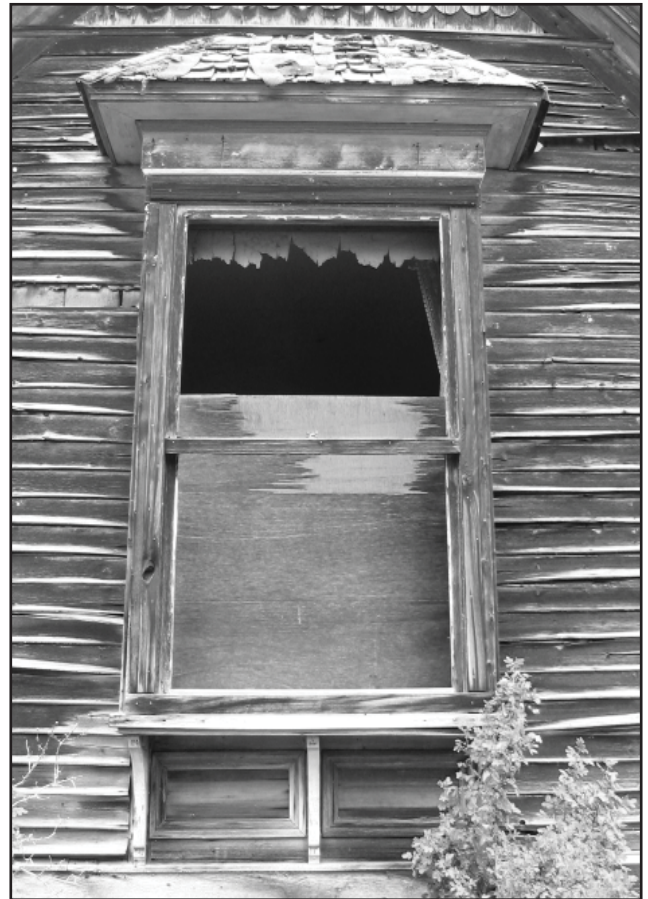
Image 11: Badly damaged historic window in need of new glazing and wood repair.
