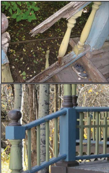
Image 7 & 8: Damaged wood porch railing with missing balustrade (top). Using historic photographs the original balustrade was recreated (bottom).
