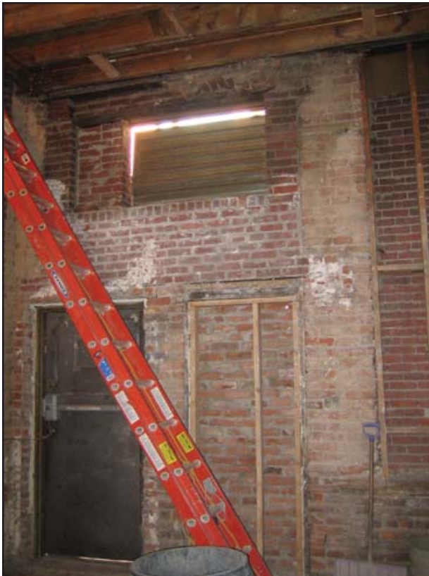
Image 6: Rear brick wall of the Red Onion. Note the different brick and mortar patches.
