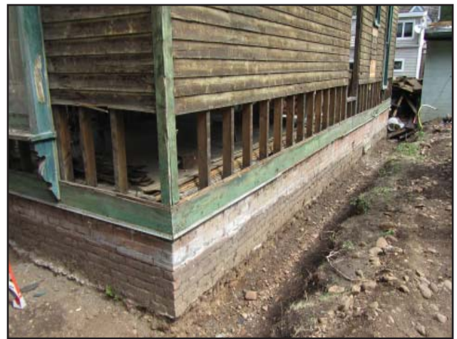
Images 14 &15: Historic home getting prepared to be relocated (top). A detail of the original foundation and documentation of foundation exposure and style (bottom).
