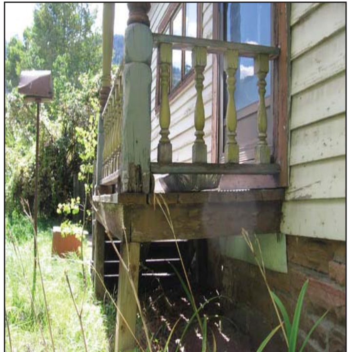
Image 12: Historic side porch with water damage and structural deterioration.
