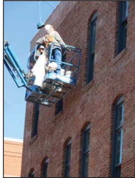
Image 5: Working on the Hotel Jerome brick restoration project. Note the size and color of brick and consistency of the mortar application.
