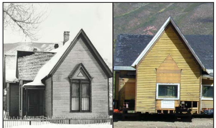
Image 9 & 10: A historic photograph (left) used in conjunction with ghost lines on the residence (right) to restore wood details and openings.
