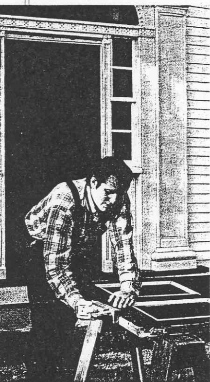
Final trimming on the bottom of the door to fit the new sill.
