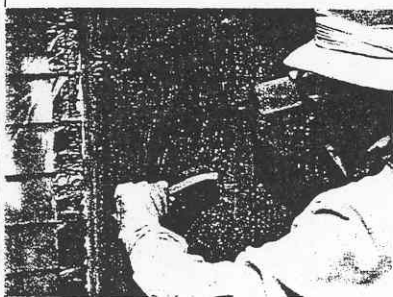
An alcohol rinse removes the last residue of chemical remover while masking protects the adjacent surface.
