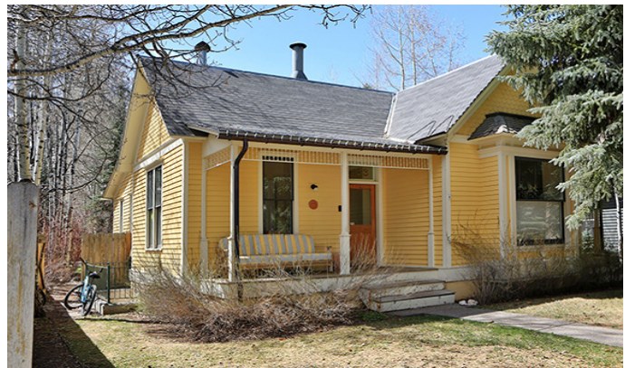
These new chimney vents are consistent with the building type, located behind the ridge line, and a dark color.
