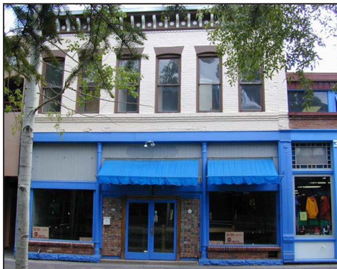
Before: Window and door openings filled in with non-historic materials.
