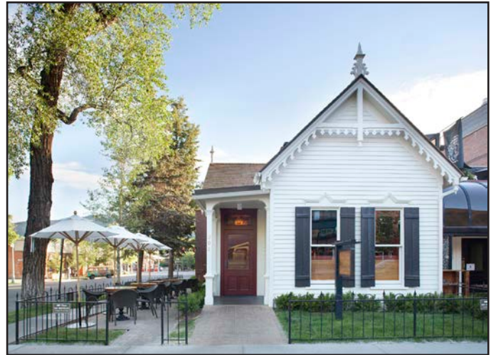
A subtle ramp eliminates the need for a step onto this historic porch and therefore meets accessibility requirements.
