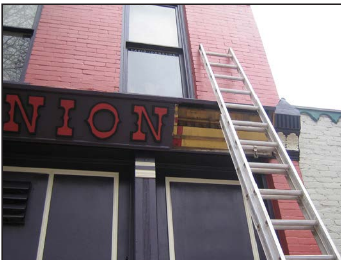
Before: A sign was installed overtop of the original decorative molding.
