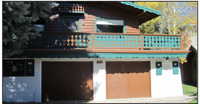
Broken balusters within this railing were carefully replicated.
