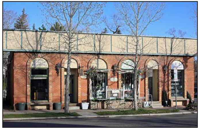
After: A cornice has been installed over the original brick.
