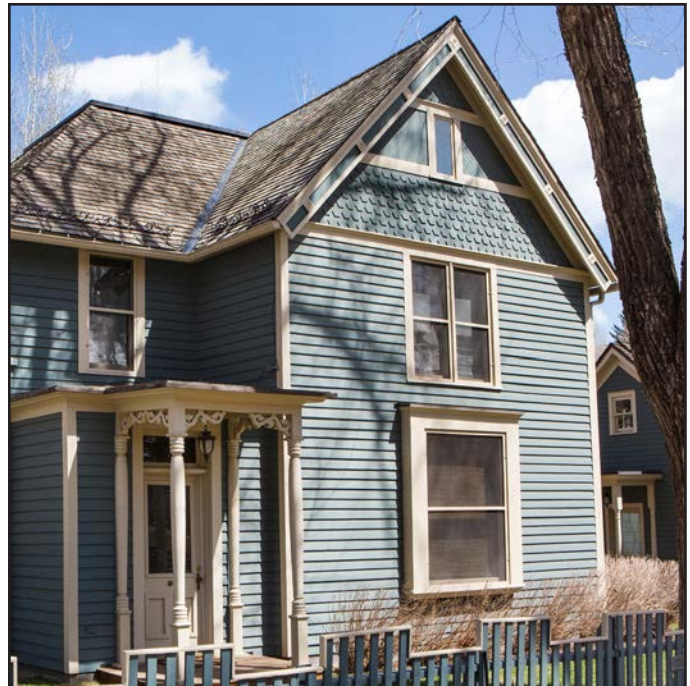
Exterior mounted wood storm windows.
