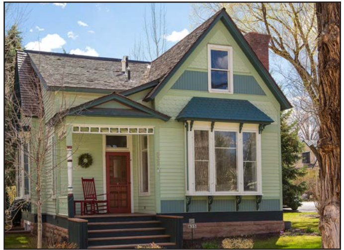
The original sandstone was used as a veneer on this foundation after a new basement was built.
