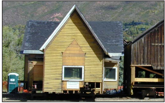
Before: Look for evidence of original openings and restore.
