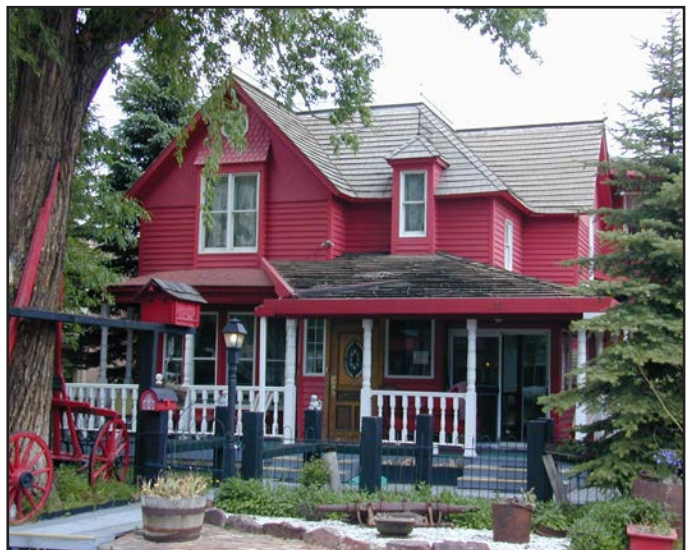
Before: A historic porch where the original posts and details were replaced with an inaccurate design.
