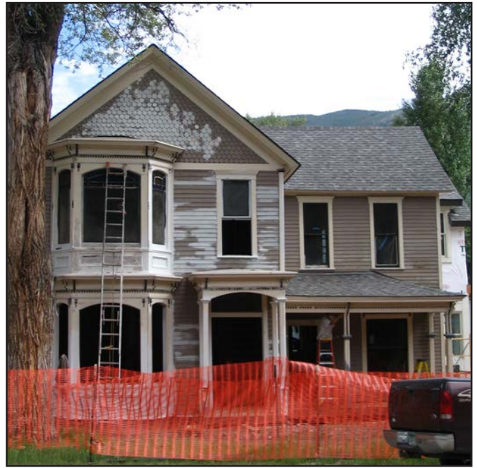
Repair of historic siding in preparation for new paint.
