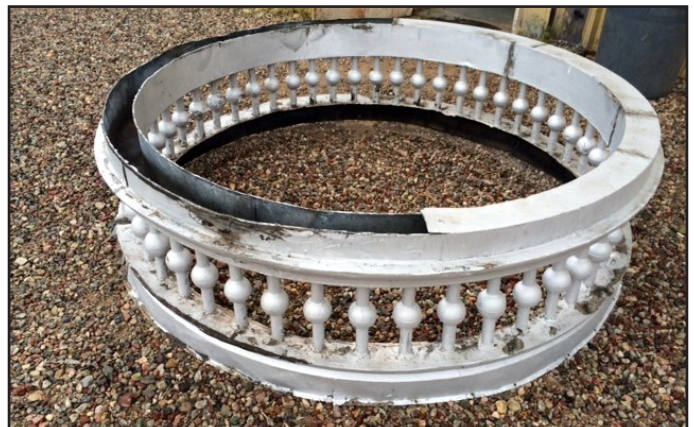
A portion of the metal crown on the Elks Building was missing and needed to be replicated.
