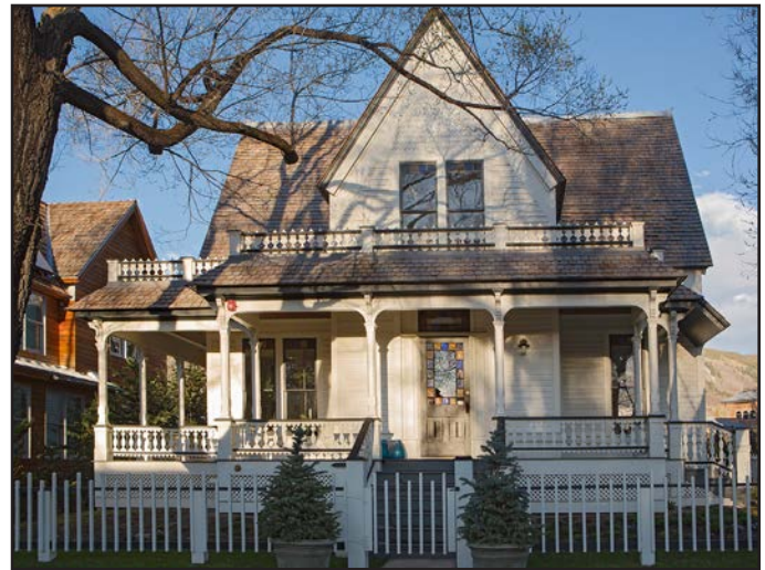
After: The same house after non-historic siding materials were removed to expose original clapboard.
