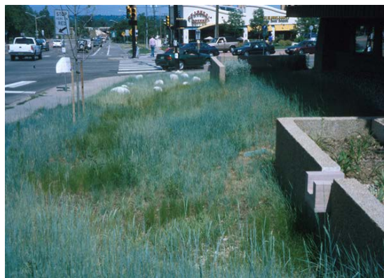
Figure 8.17 A shallow grass swale collects runoff from roof downspouts and adjacent pavement. The flush curb allows sheet flows into the swale.
