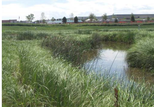
Figure 8.38 Man-made Constructed Wetland Channels can enhance the ecological value of open spaces while treating and managing urban runoff.
