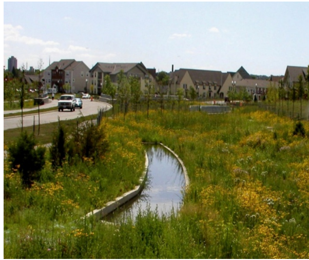
Figure 8.46 This larger Bioretention area manages stormwater runoff for a medium density residential neighborhood. The forebay sediment trap (in the foreground) is located at the outlet of the storm sewer to trap settlement larger
