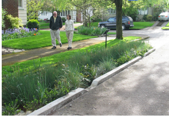
Figure 8.5 Typical Residential Street Biofiltration Planter Slotted curbs allow stormwater runoff into biofiltration planters.
