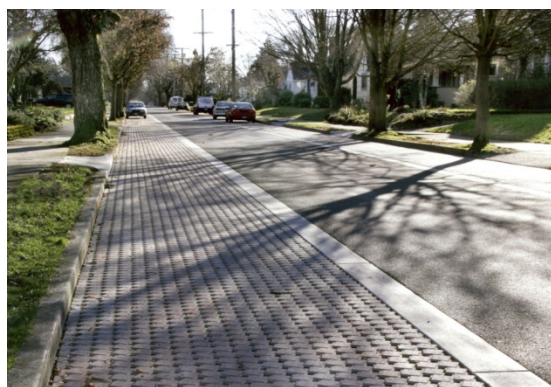
Figure 8.27 Modular block permeable pavement is used for an on-street parking lane on this residential street.
