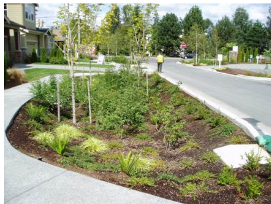
Figure 8.47 Rain gardens are used to collect and filter stormwater runoff. As seen in the examples above they can be planted in a variety of areas with a wide variety of plant life from flowers and grasses to trees.
