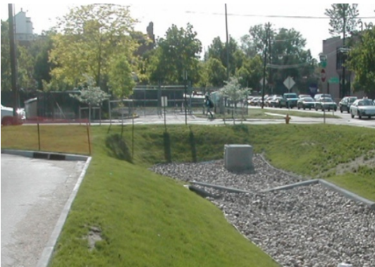
Figure 8.55 Typical Extended Detention Basins are normally designed at the outlet of storm sewers—"end of pipe". EDB's can manage large volumes of stormwater runoff utilizing a single BMP facility. This EDB has steep side slopes and a deep ponding depth and therefore limits the range plant species that can survive in this environment.
