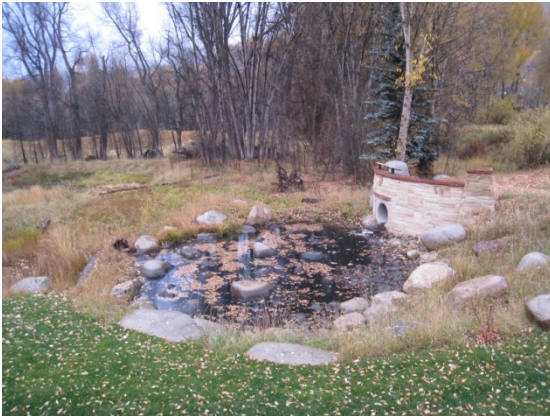
Figure 8.64 Large wetlands can provide regional stormwater treatment and detention as well as create valued habitat. The forebay and pond, shown here, dissipates stormwater velocities and allows larger particles to settle
