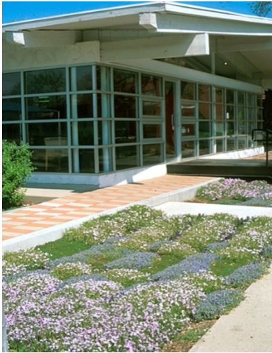
Figure 8.45 Bioretention planters can be used to treat stormwater runoff from the building site and roof, as well as being attractive planting areas or flower gardens
