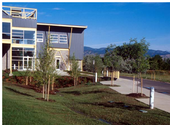
Figure 8.18 Native grass species can be utilized in swales when the longitudinal slope of a swale is flat-- less than 0.5 percent
