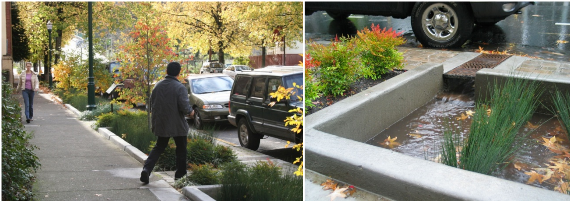
Figures 8.6 and 8.7 Typical Urban Street Biofiltration Planters Curb cuts, and chases, with metal grated covers, convey stormwater runoff from the curb to biofiltration planters located along streets.
