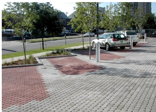
Figure 8.26 Modular block permeable pavement in this small parking lot allows runoff from roof downspout, promoting infiltration and reducing the overall storage volumes for the site.
