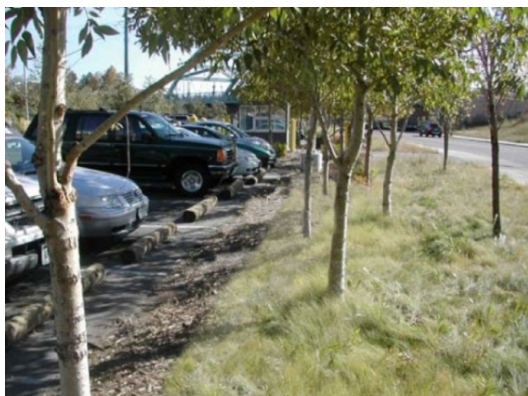
Figure 8.21 A gravel mulch band next to the traps sediment before it enters the grass buffer.
