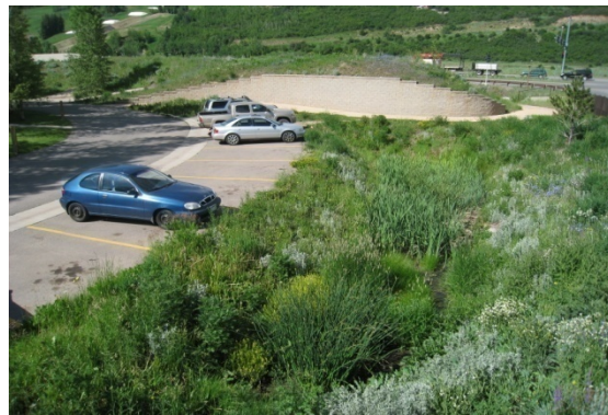
Figure 8.56 This Extended Detention Basin is spread out over the length of the parking lot, has minimal side slopes, and a shallow ponding depth. This design criteria allows this basin to utilize a greater plant species diversity than that of Figure 8.55
