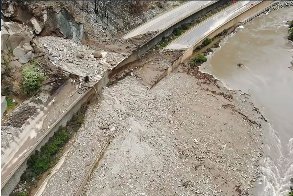
An aerial image of damage from mudslides to I-70 in Glenwood Canyon in Colorado. Colorado Transportation Department
