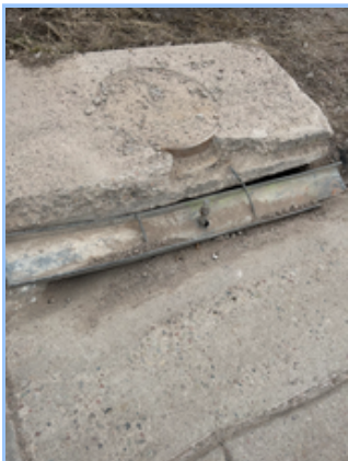
Broken Stormwater Inlet
