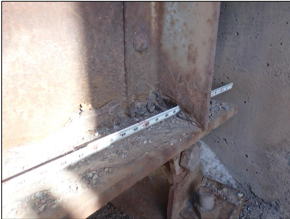
Figure 33: Corrosion Hole in Base of Bearing Stiffener – Girder F at Abutment 6
