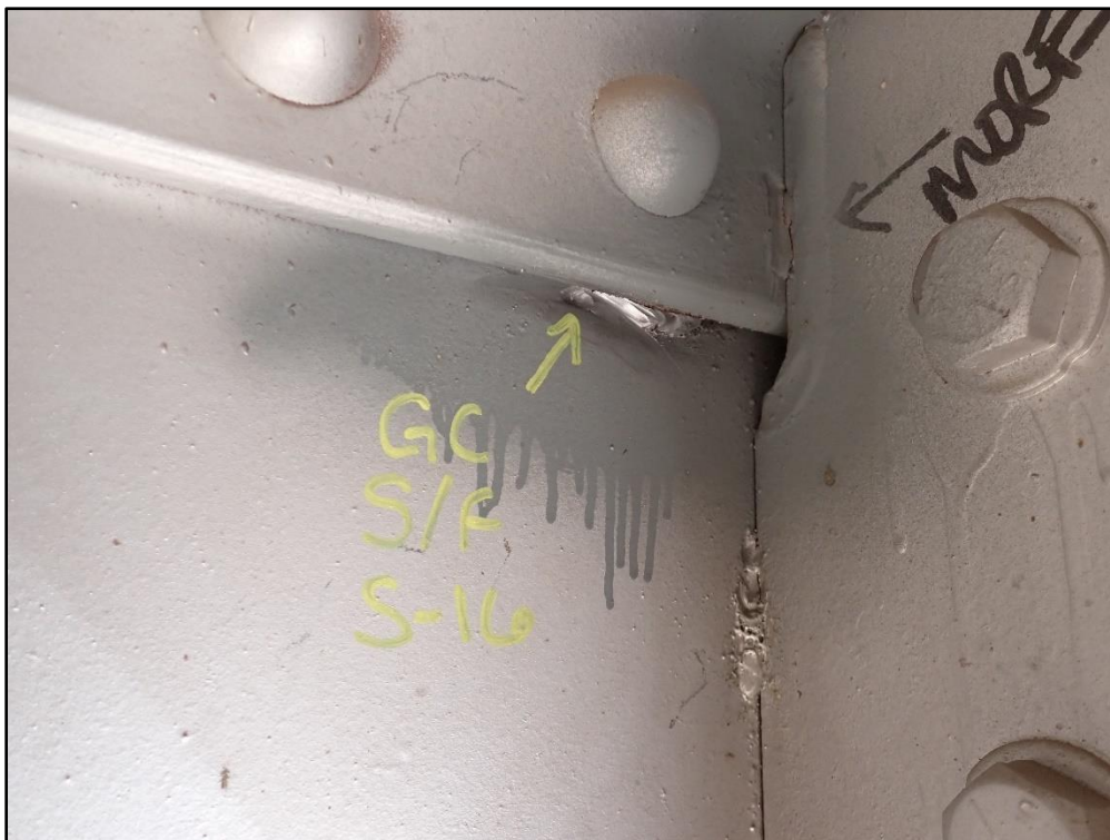
Figure 20: Partially Ground Out Tack Weld – Girder C South Face – Girder Top Flange to Web At Stiffener 16
