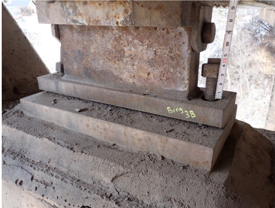
Figure 24. Loose Anchor Bolt Nuts – Typical at All Bearings
