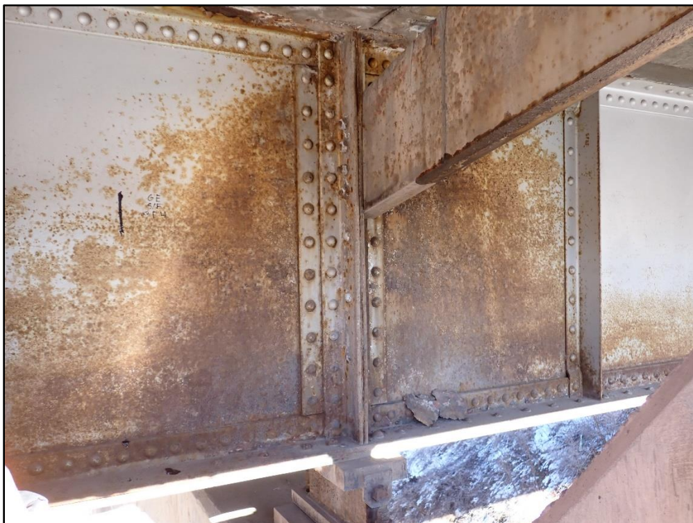
Figure 24: Typical Surface Corrosion of Interior Girder at Pier – Girder E South Face at Pier 4
