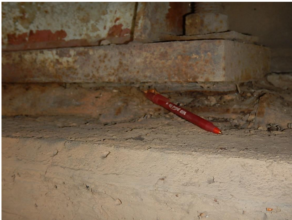
Bearing Loss Due to Missing Grout Pad Under Bearing 6B
