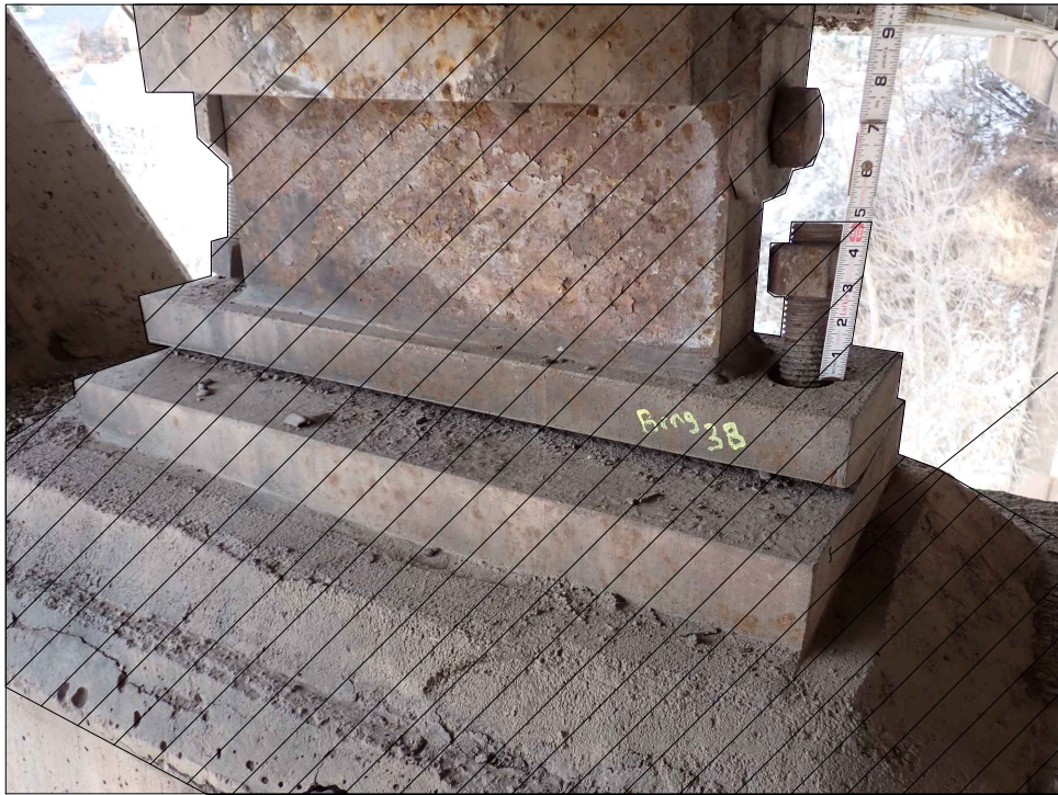
TYPICAL EXPANSION ROCKER BEARING AT PIER
