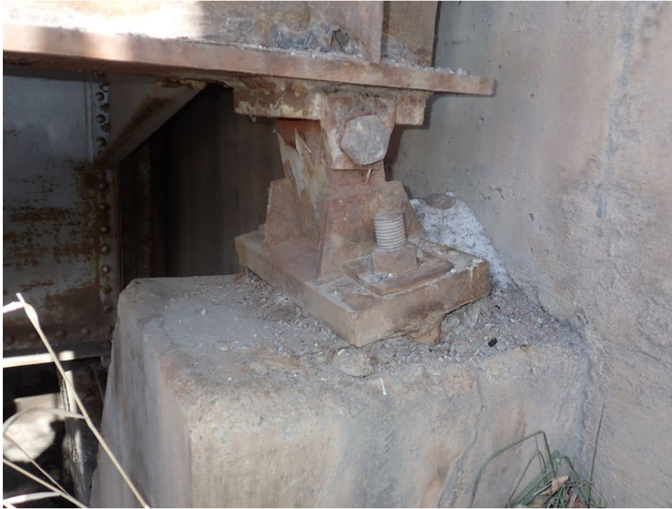
Figure 23. Impending Spall in the Bearing Pedestal at Bearing 6A at Abutment 6
