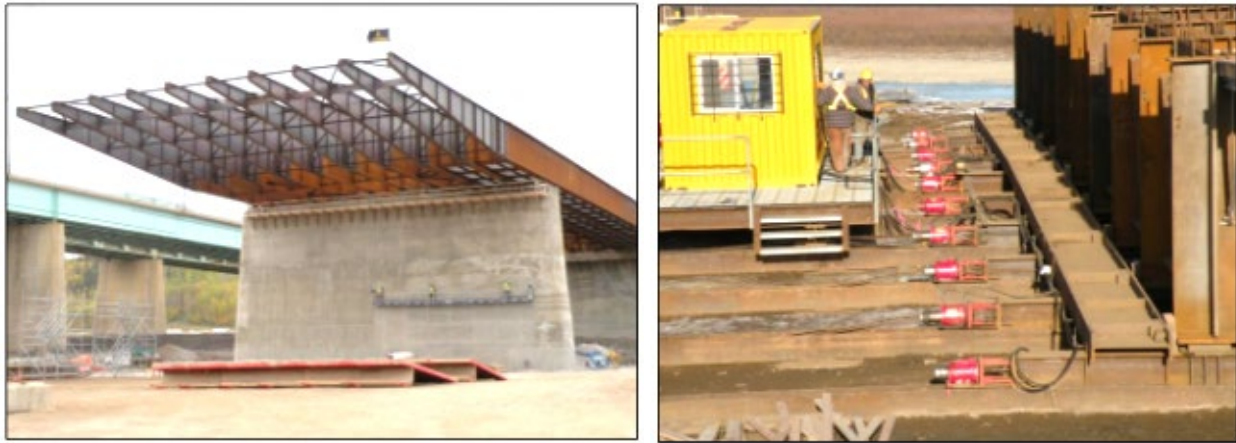
Figure 48. Incremental Steel Bridge Launch at the Athabasca River Bridge
