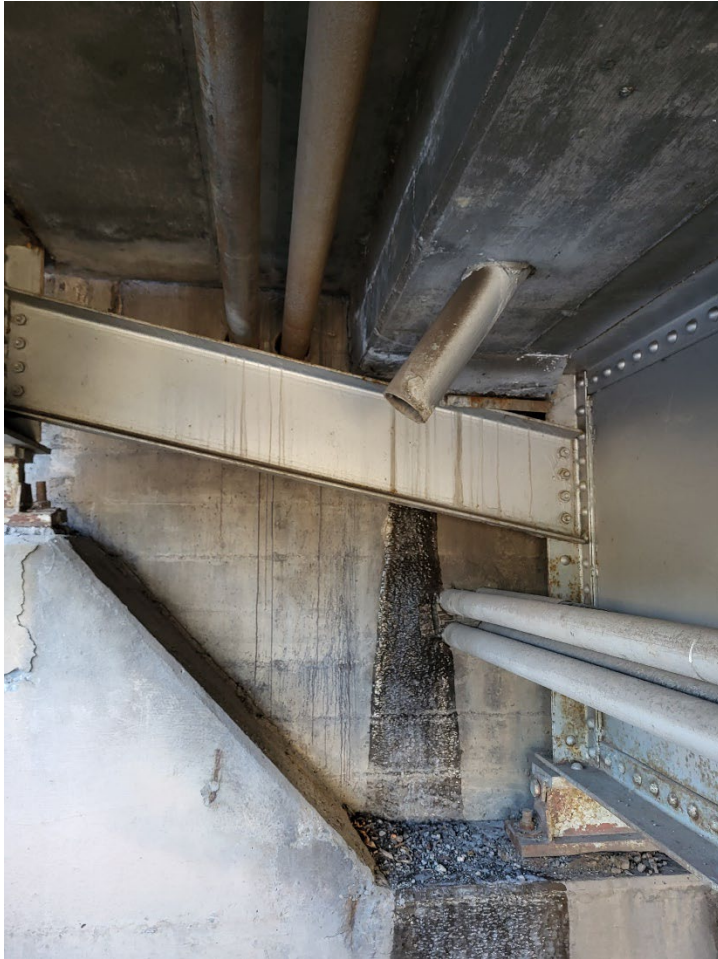
Figure 29. Light Scale, Delamination and Water Staining at Abutment 6
