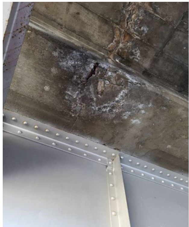
Figure 12. Deck Concrete Spall with Exposed Rebar
