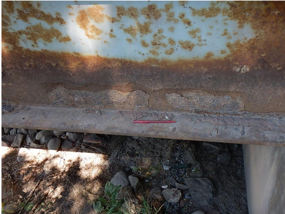
R3 - R4 Corrosion of Girder 5F near Abutment 6
