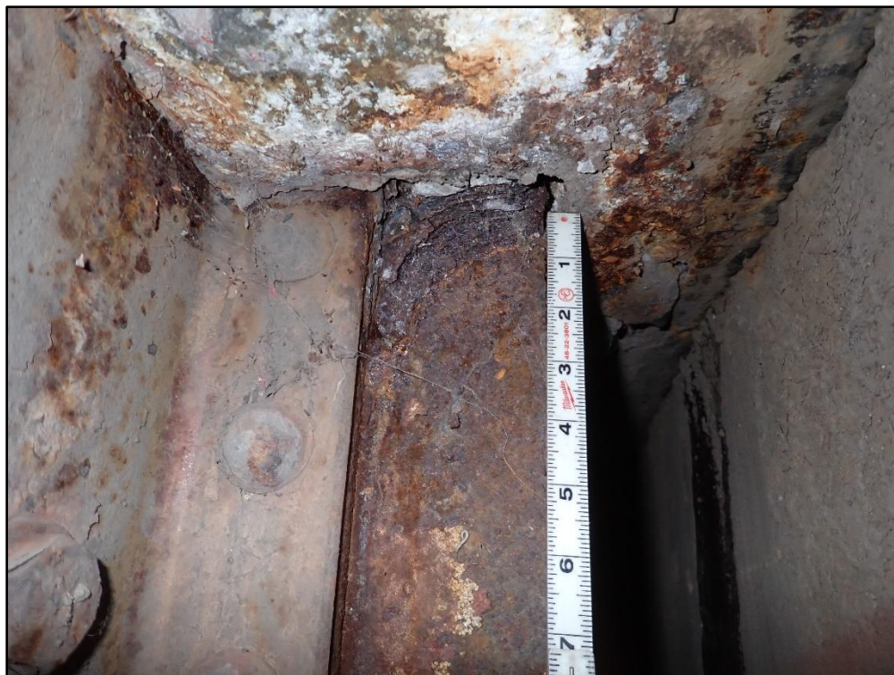
Figure 26: Laminar Corrosion of Girder E End at Abutment 6
