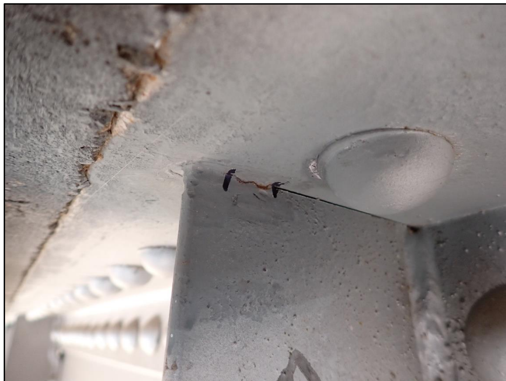
Figure 10: NSA Cracked Tack Weld – Girder B South Face – Stiffener 19 to Horizontal Leg of Top Flange Angle
