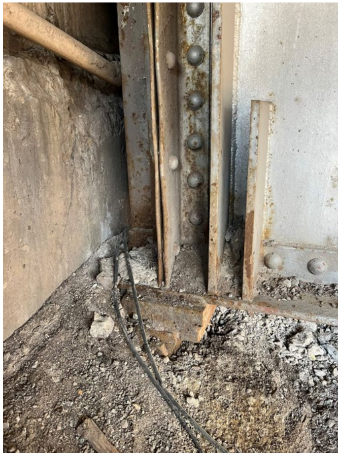
Figure 21. Rocker Bearing Covered in Dirt – Typical at Abutment 1
