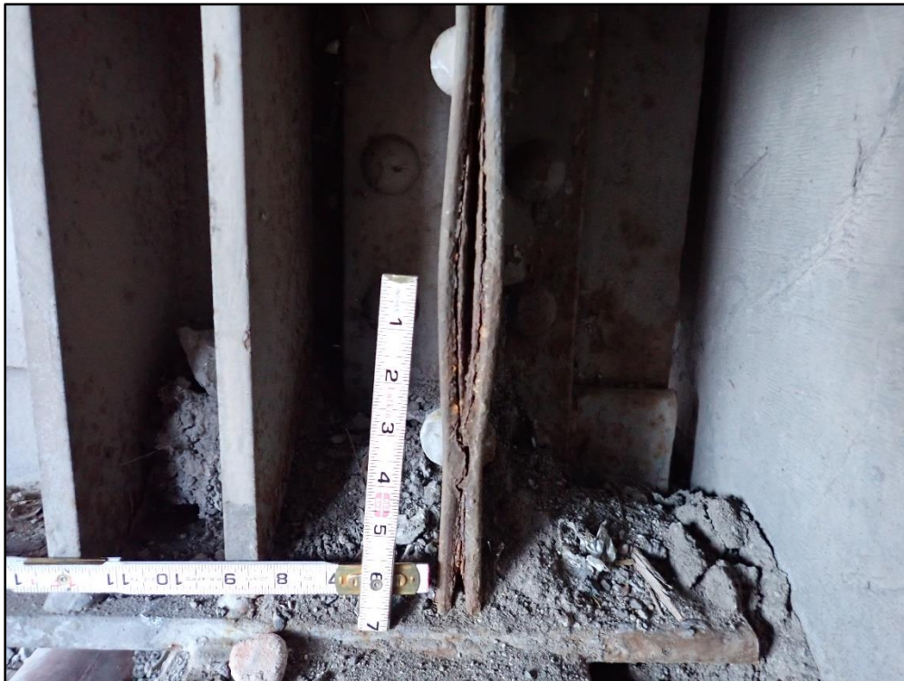
Figure 28: Typ. Pack Rust between Bearing Stiffeners of Int. Girders at Abut. – Girder B N. Face at A1 – Stiffener 1
