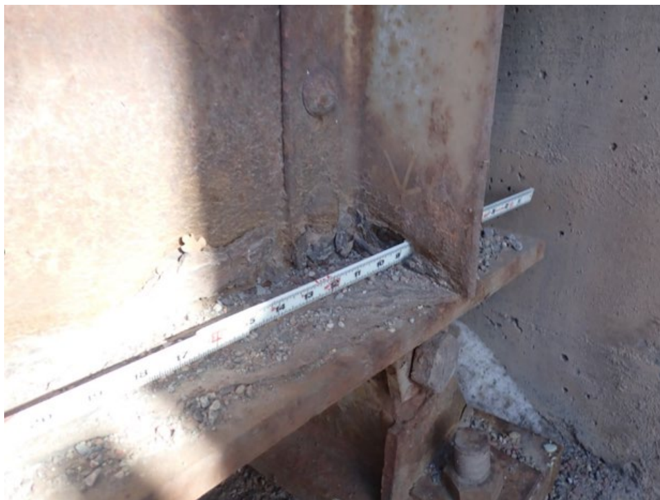
Figure 18. Section Loss in Base of Bearing Stiffener – Girder F at Abutment 6
