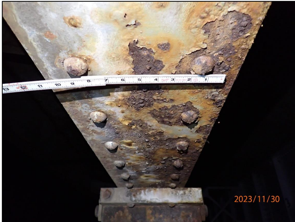
Figure 25: Surface Corrosion and Minor Pitting in Bottom of Bottom Flange of Girder E at Pier 4
