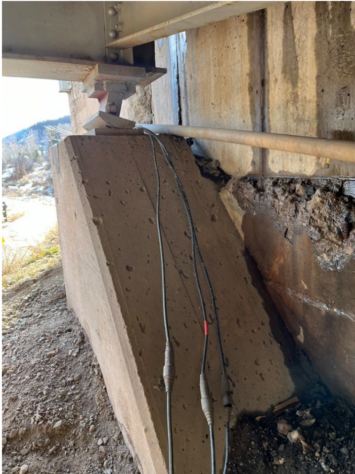
Figure 28. A Portion of Abutment 1 Backwall Was Removed During Previous Construction
