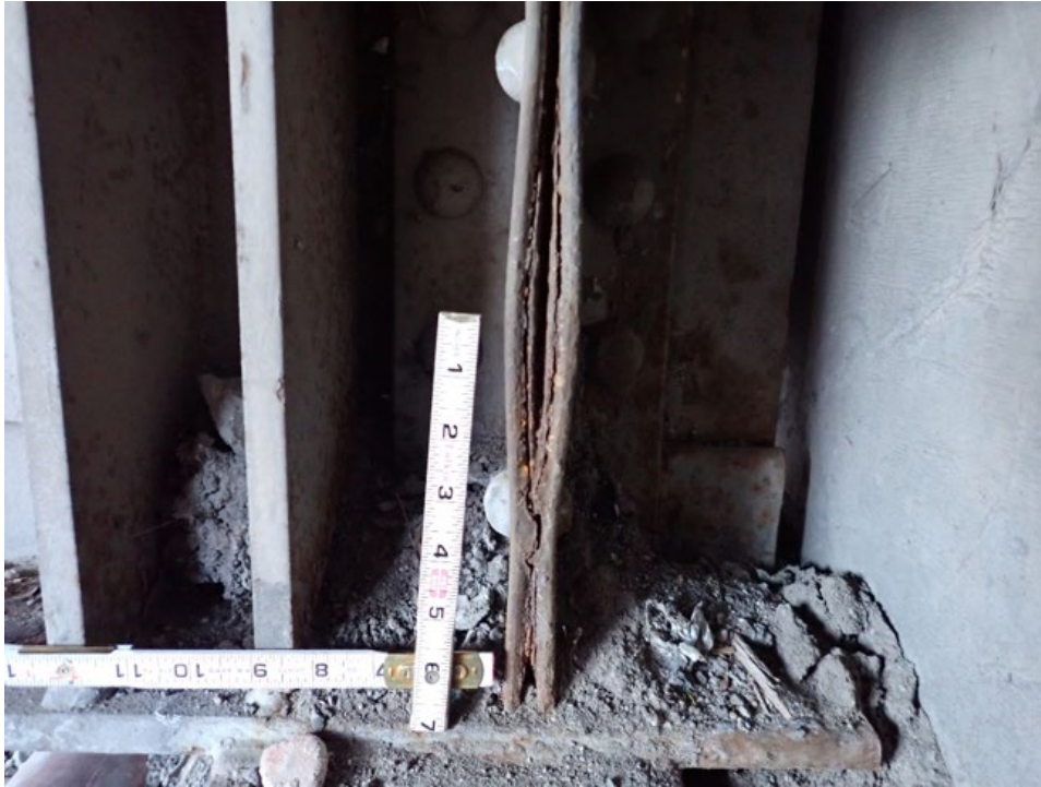
Figure 19. Pack Rust Between Bearing Stiffeners of Interior Girder at Abutment 1
