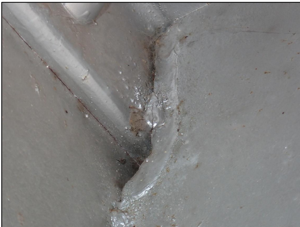
Figure 14: NSA Cracked Tack Weld – Girder E North Face – Stiffener 107 to Vertical Leg of Top Flange Angle
