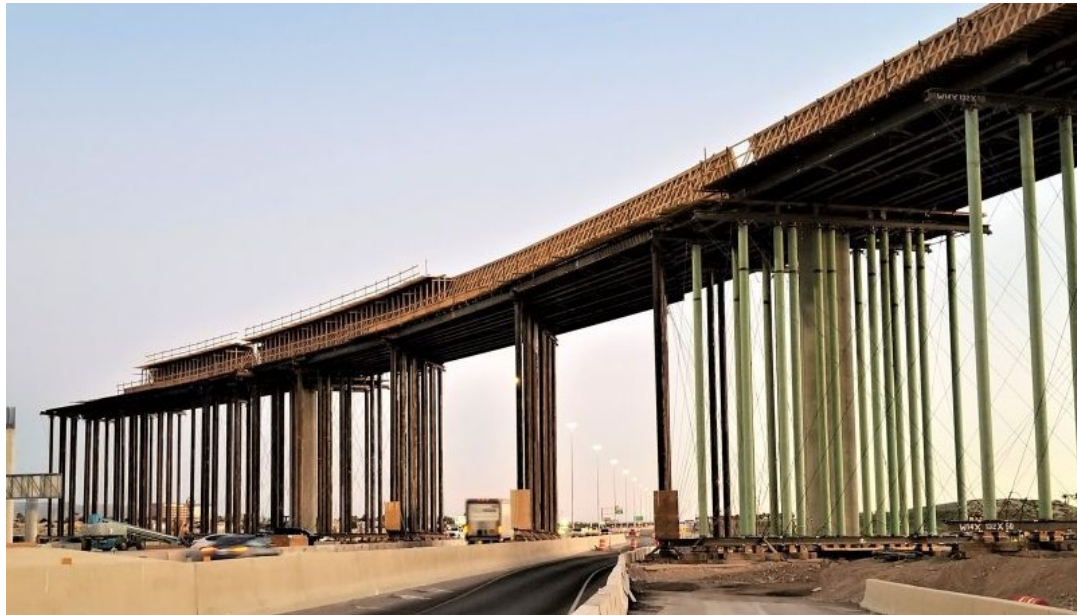
Figure 38. Example Falsework Photo for Cast-in-place Concrete Construction
