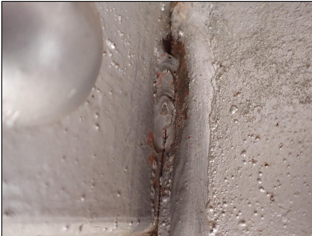
Figure 13: NSA Cracked Tack Weld – Girder D North Face – Stiffener 97 to Vertical Leg of Top Flange Angle
