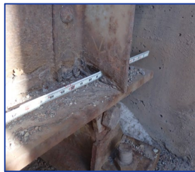
Hole in girder stiffener
