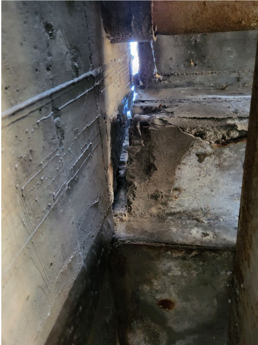
Figure 30. Inadequate Joint Seal at Abutment 6
