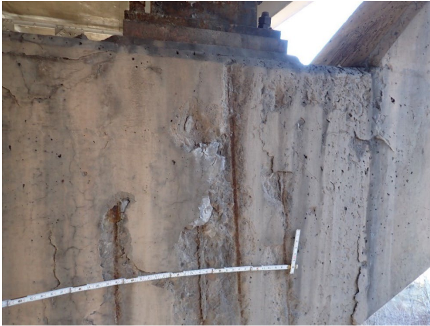
Figure 27. Light Scale Cracking at Pier Cap – Typical at All Pier Caps
