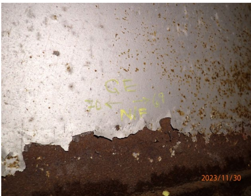
Figure 20 Failure of Protective Coating - Typical on All Steel Sections
