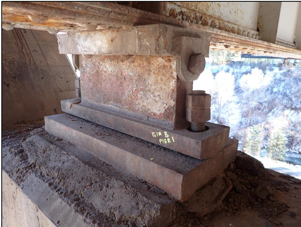
Figure 35: Typical Surface Corrosion of Bearing at Pier – Girder B at Pier 1
