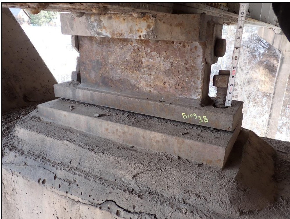
Figure 36: Typical Anchor Bolt Nut Backed Out and Missing Lock Nut – Girder B at Pier 2
