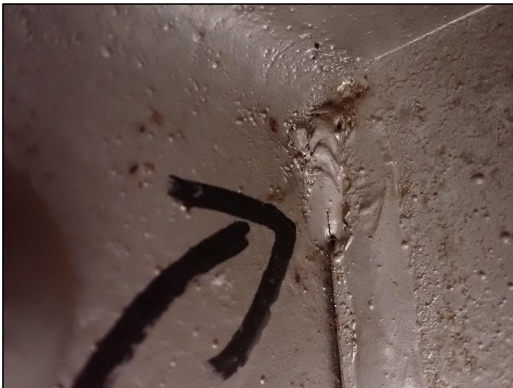
Figure 12: NSA Cracked Tack Weld – Girder C North Face – Stiffener 105 to Vertical Leg of Top Flange Angle
