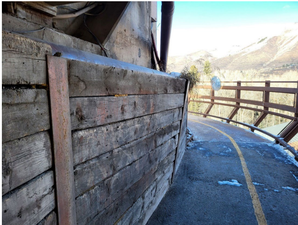
Figure 31. Movement of Timber Retaining Wall at Abutment 1
