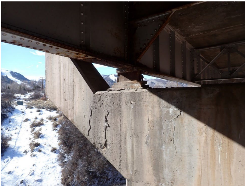
Figure 27. Light Scale Cracking at Pier Cap – Typical at All Pier Caps
