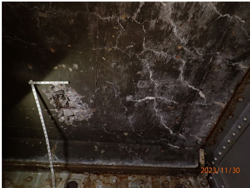
Figure 13. Deck Concrete Spall with Exposed Rebar
