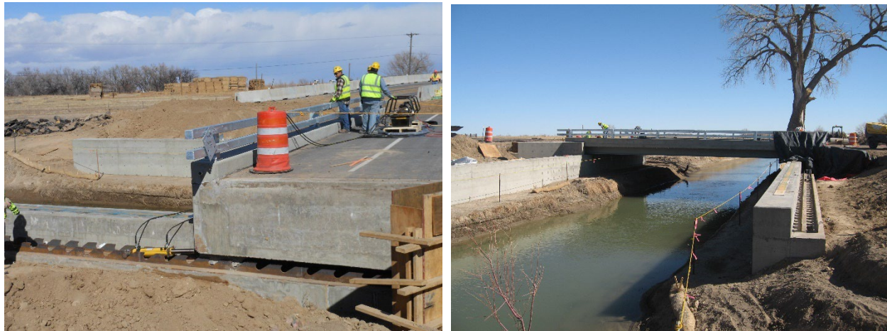
Figure 49. Slide-in Bridge Construction at the Colorado Department of Transportation State Highway 266 over Holbrook Canal Bridge
