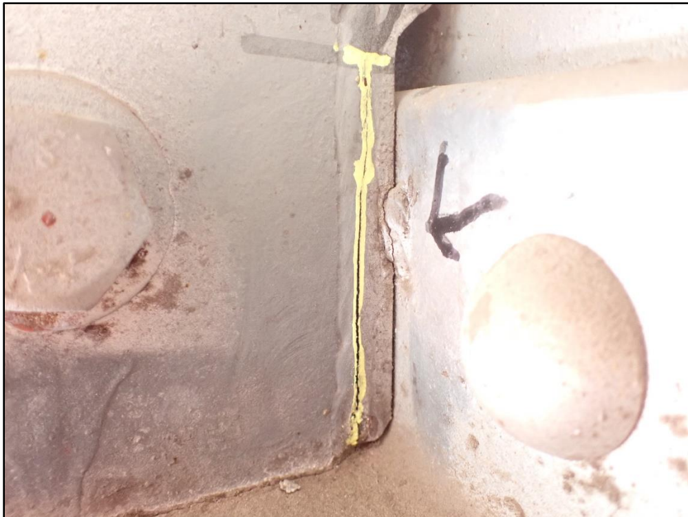
Figure 22: Fractured Stiffener 16 Weld – Girder C North Face at Bottom – Right
