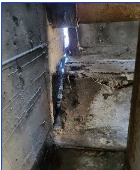
Inadequate joint seal at Abutment 6
