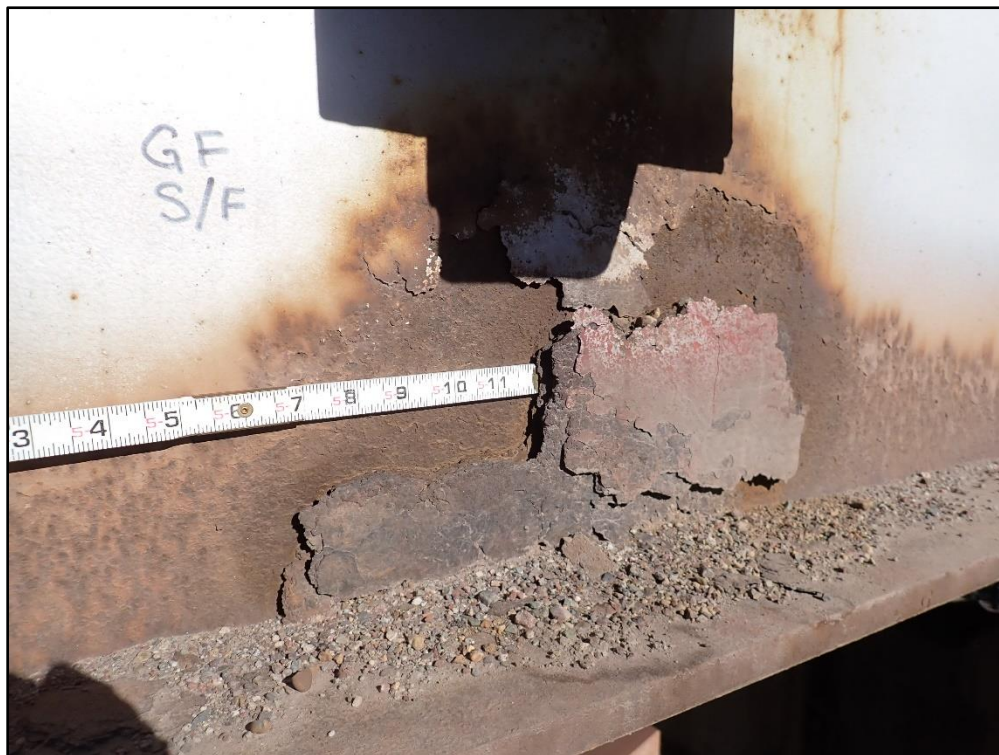
Figure 32: Laminar Corrosion in Web of South Exterior Girder F
