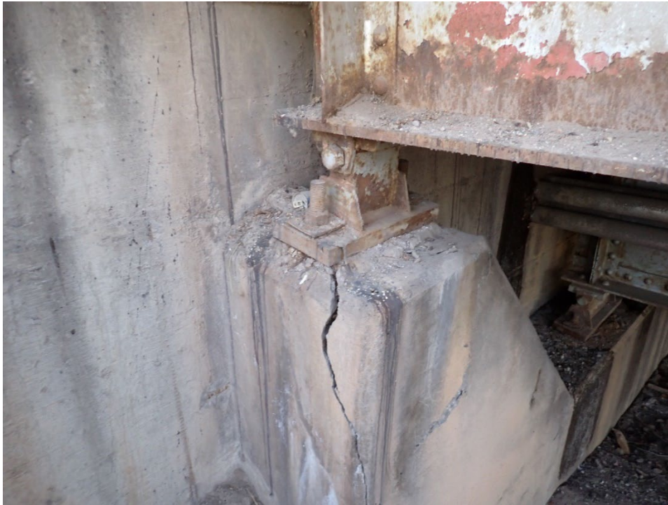
Figure 23. Impending Spall in the Bearing Pedestal at Bearing 6A at Abutment 6
