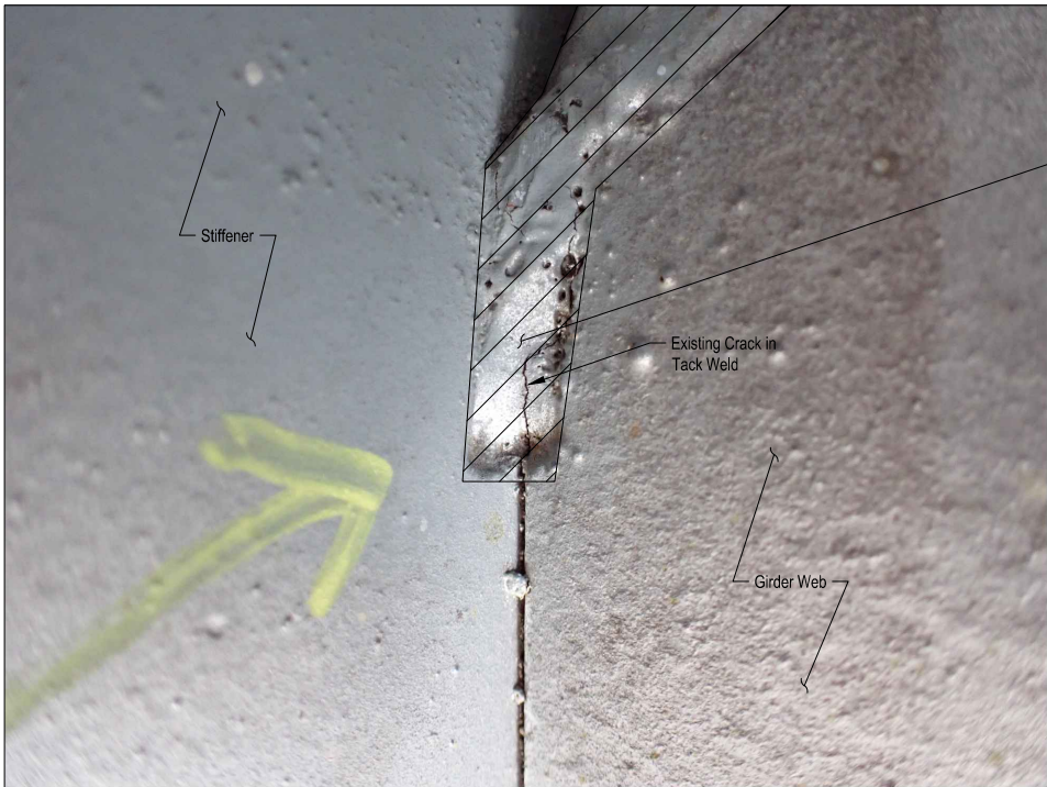
TYPICAL STIFFENER TACK WELD
