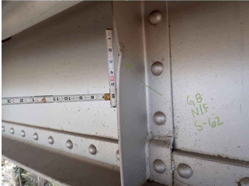
Figure 17. Deflection of Stiffener at North Face of Girder B
