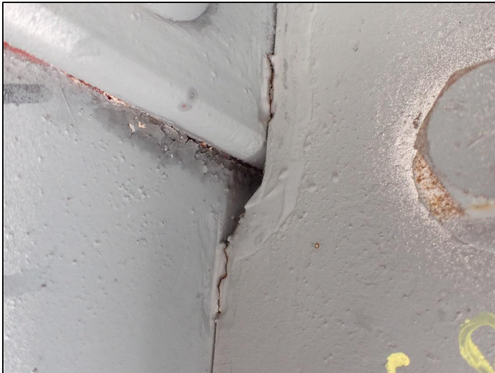
Figure 16: SA Cracked Tack Welds – Girder B South Face – Stiffener 41 to Vertical Leg of TF Angle and Web
