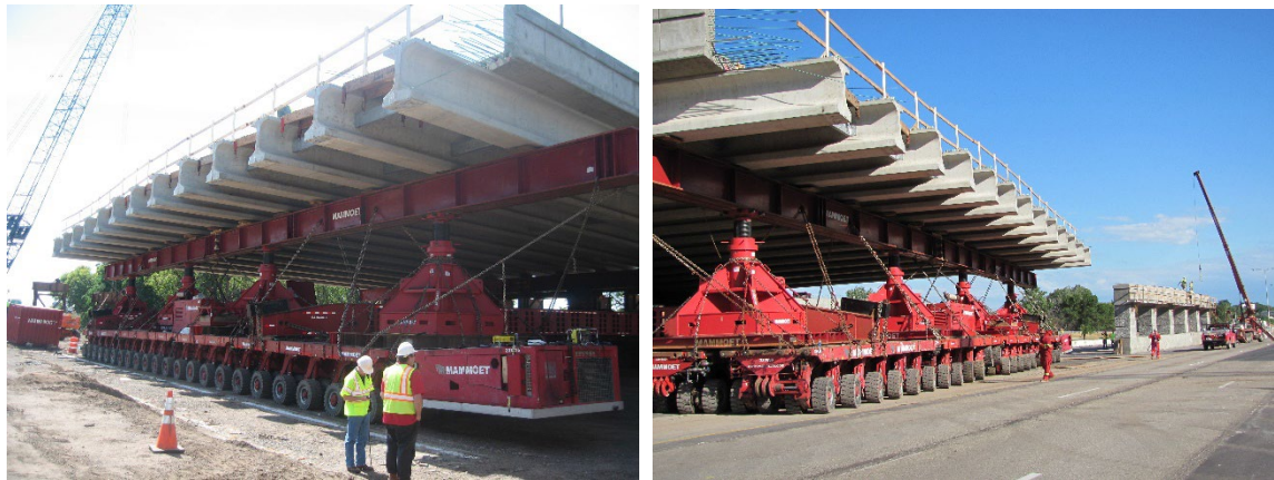
Figure 47. Self-propelled modular transporter construction on Minnesota Department of Transportation Maryland Avenue Bridge
