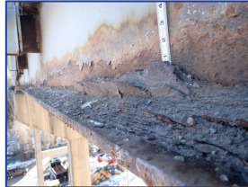
Considerable girder corrosion
