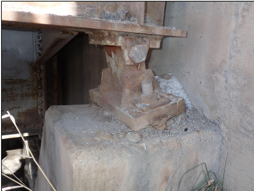
Figure 38: Tilted Bearing of Girder F at Abutment 6
