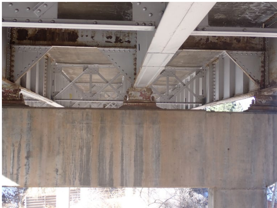
Figure 25. Surface Corrosion of C-Channel Diaphragms – Typical at All Diaphragms
