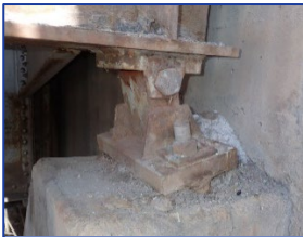
Bearing movement at Abutment 6
