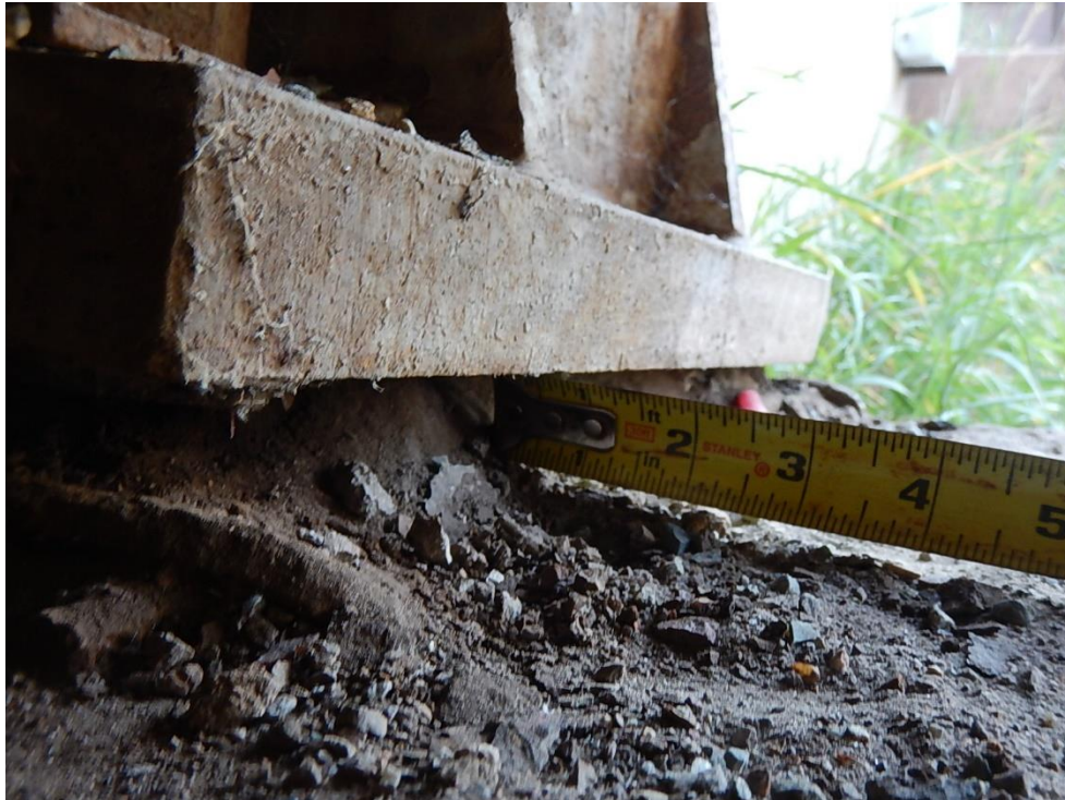
Broken Bearing Pad under Bearing F at Abutment 6 15 Percent Bearing Loss
