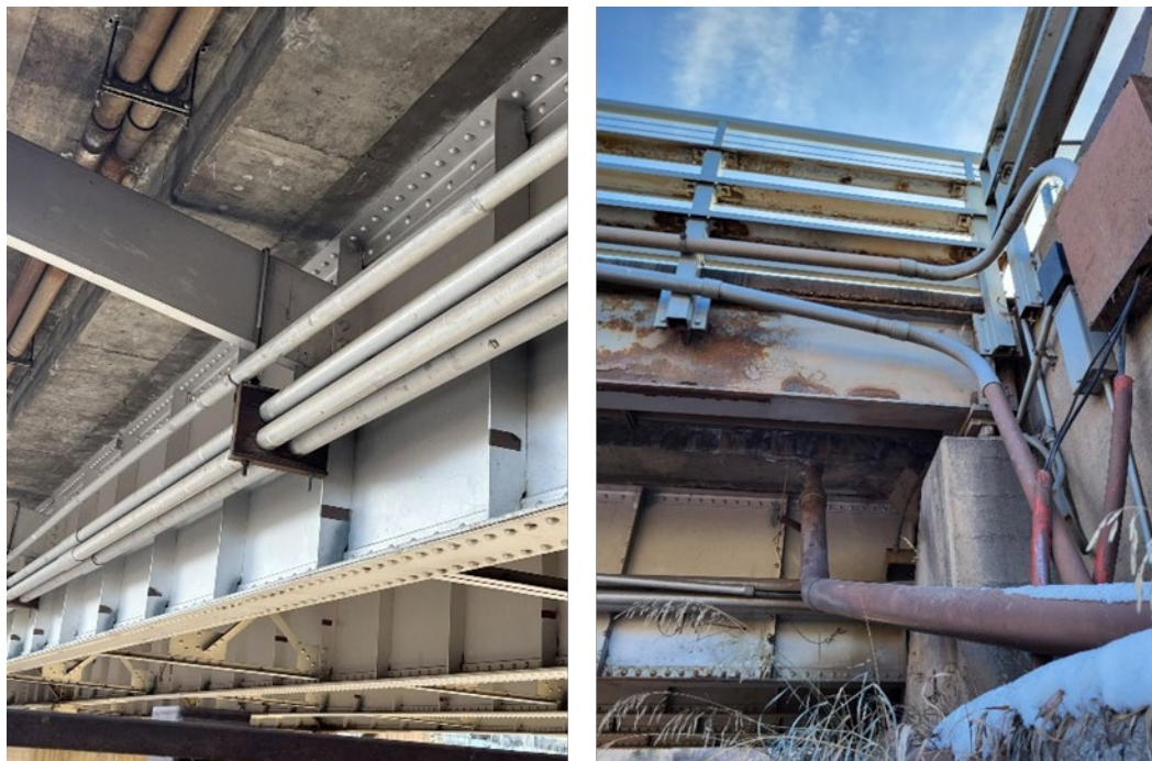
Figure 8. Utilities Along Bridge and Connection at Abutment 1
