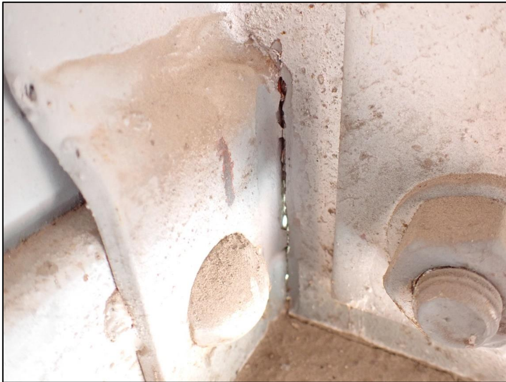
Figure 21: Fractured Stiffener 16 Weld – Girder C North Face at Bottom - Left
