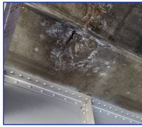
Deck concrete spall with exposed rebar
