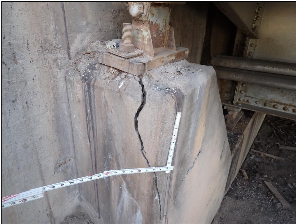
Figure 37: Impending Spall of Bearing Pedestal of Girder A at Abutment 6
