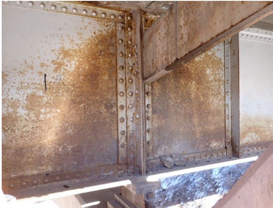
Figure 16. Typical Surface Corrosion of Interior Girder – Girder E South Face at Pier 4
