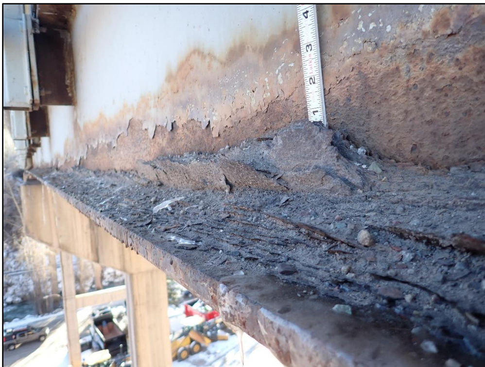
Figure 30: Laminar Corrosion in Web and Top of Bottom Flange of North Exterior Girder A
