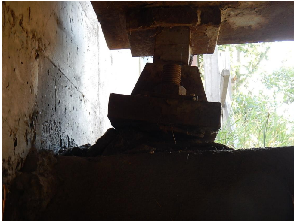
Bearing 6F is Tilting to the Rear
