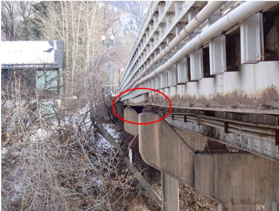
Figure 15. Girder F Sagging Near Mid-span
