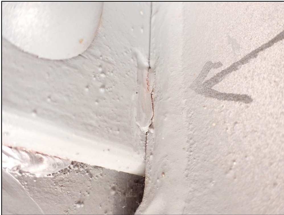
Figure 15: SA Cracked Tack Weld – Girder C South Face – Stiffener 16 to Vertical Leg of Top Flange Angle
