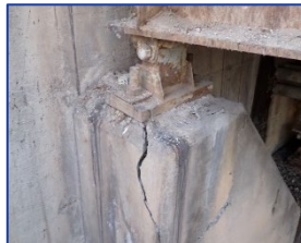
Bearing pedestal crack
