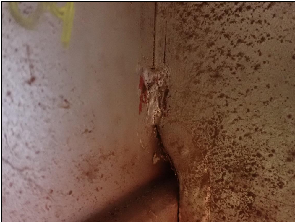
Figure 18: NSA Cracked Tack Weld – Girder C North Face – Stiffener 109 to Web
